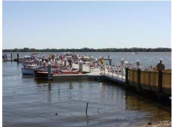
One of the new docks at Tavares
